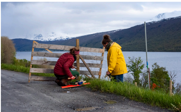
S.K. and K.K. setting up a fence installation (photo: Vidar Laksfors)
